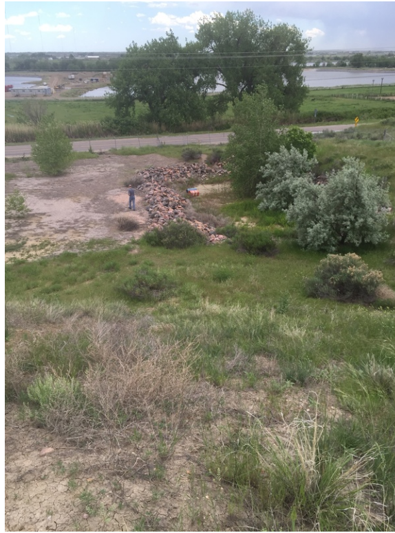
South Shooting Range Stormwater Basin
