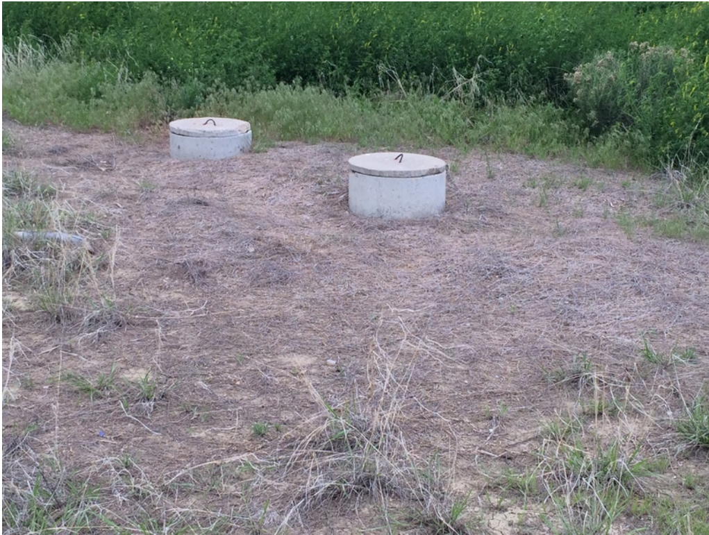
Septic tank and leach field within former skeet shooting area
