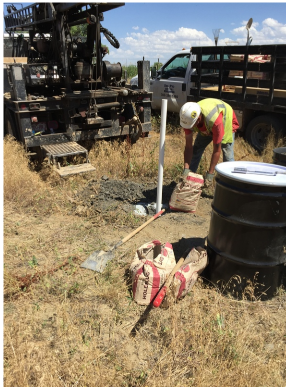
Installing groundwater monitoring wells
