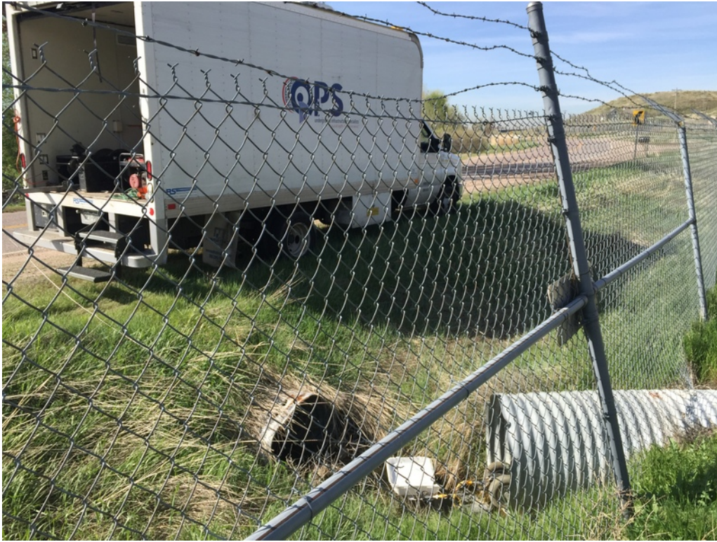
CCTV sewer video from 30" storm sewer outlet
