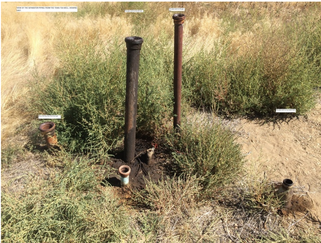
Texas Tea Well separator pipes
