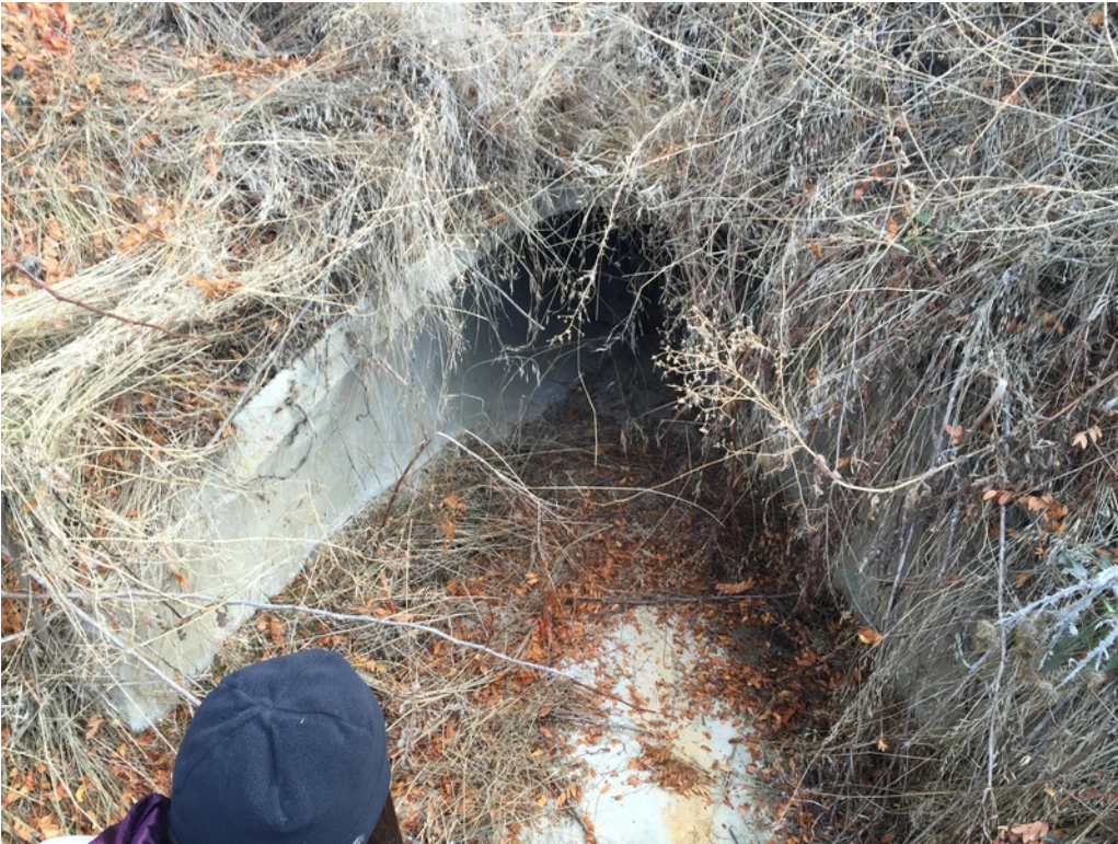
30" CMP storm sewer drainage pipe inlet
